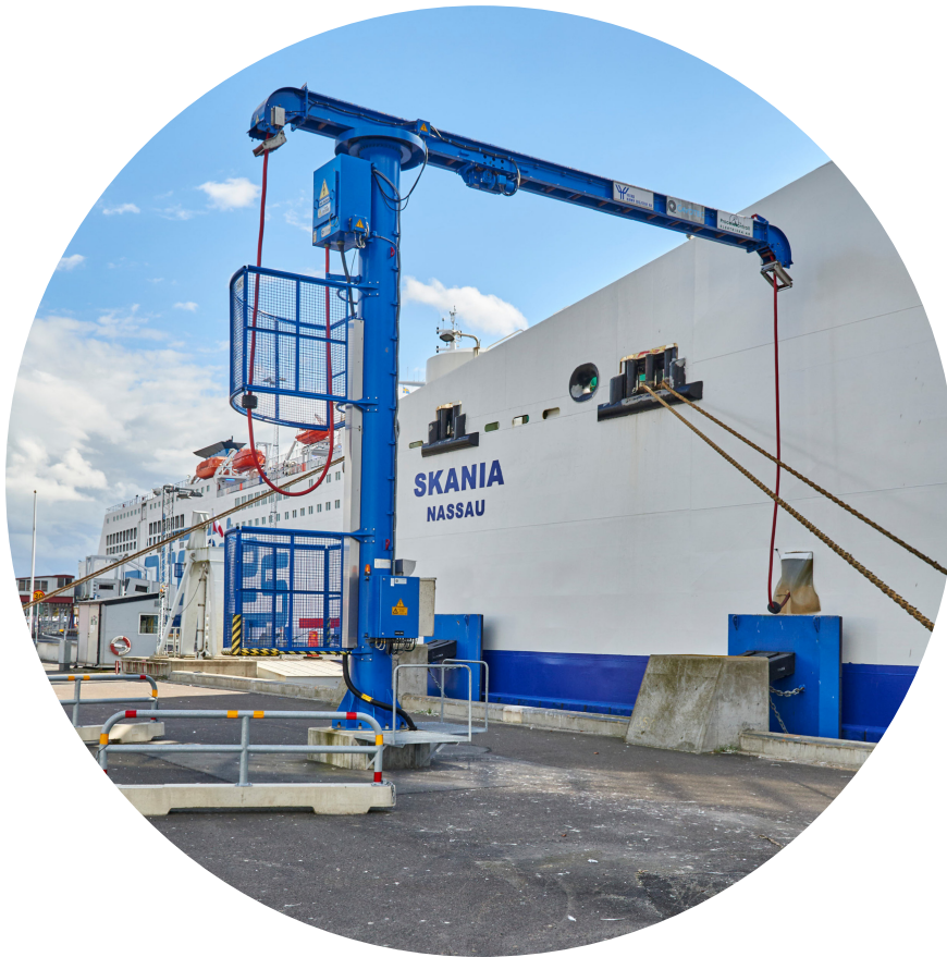
High Voltage Shore Connection 50 & 60 Hertz
